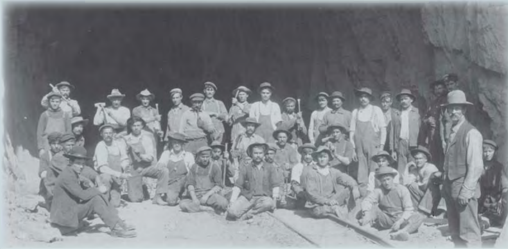
Building the Echo Canyon Railroad Tunnel for the Great Northern Railroad, May 5, 1907, Courtesy of the Western Heritage Center
